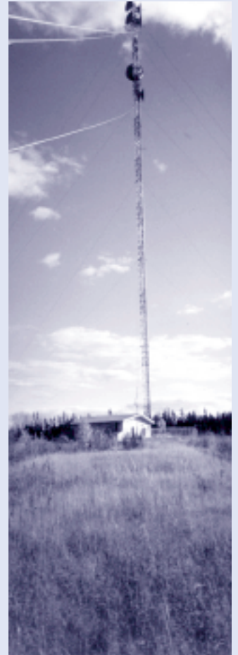
MTS maintains over 600 buildings and satellites in urban, agricultural, and isolated locations.
